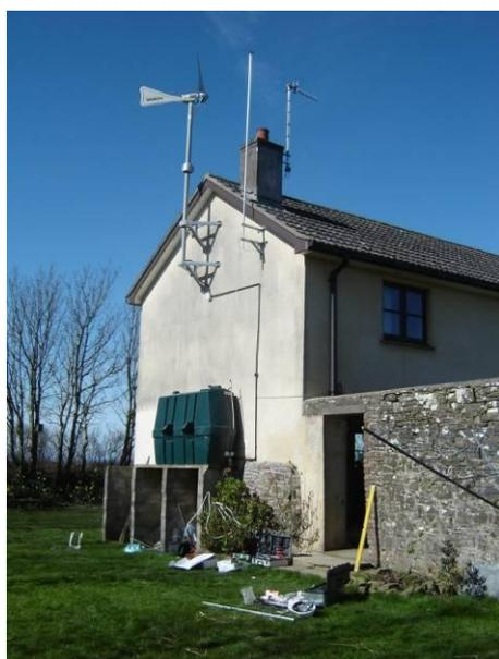
West Staddon Farm is a farm house located in north Devon close to the coast. This is the latest Windsave mounting system with a mass damper attached to the pole to reduce vibrations.
