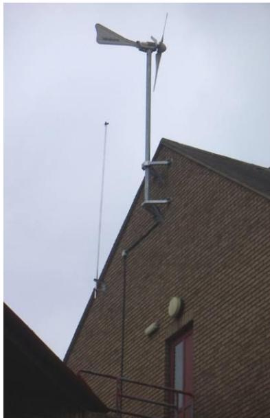
The Civic Centre is in the centre of Daventry. The wind turbine is installed on the civic centre building at about 15 meters above ground level and 2 meters above the roof line of the building.
