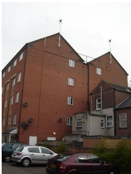
Delta Court is a four story block of flats in Nottingham. The building is on top of a hill and the turbine is mounted 3 meters above the roof line.
