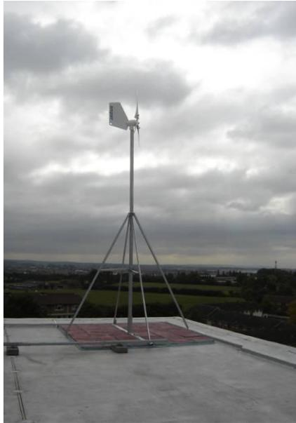
Southorn Court is a seven storey block of flats. Like on Eden Court the turbine is mounted on top of a 5 meter pole held down by ballasting the base of the mount.
