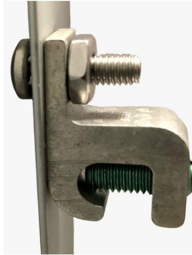
Figure 24 Installed Grounding Lug
